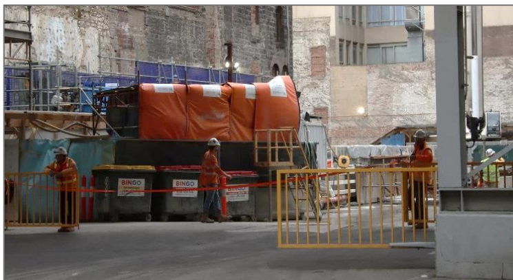
Melbourne Metro Tunnel Project
