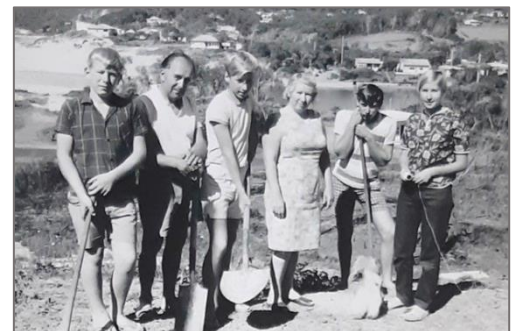
1964: Leveris family with spades, begin to build their holiday house at Copacabana Beach NSW
